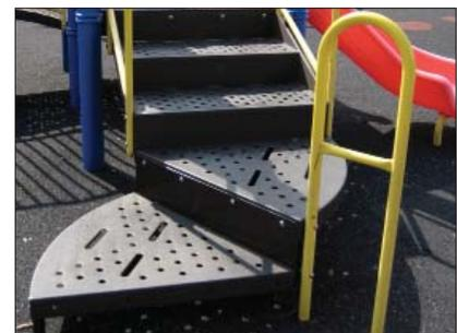
*Transfer system to connect elevated play components.*
