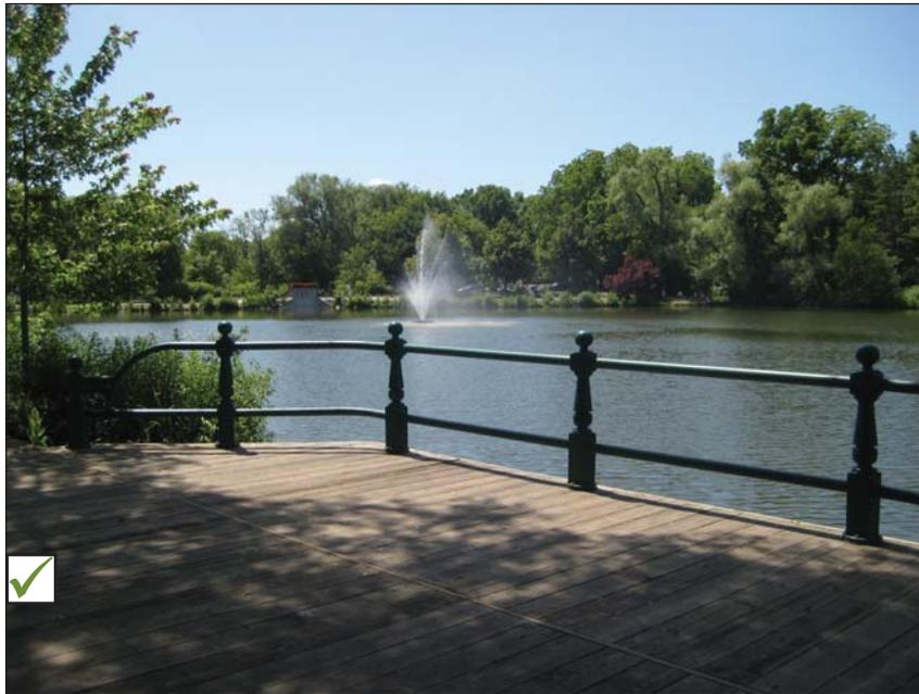
*Example of edge protection where there is a large elevation change or trail is adjacent to water feature.*
