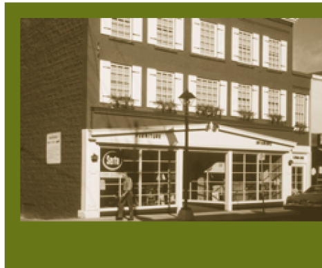
Creating a false sense of history, such as adding features based on 18 th century American architecture to a 19 th century Canadian building, is not recommended.
