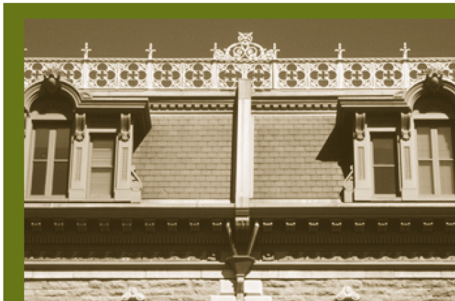
In Rehabilitation , replacing in kind an entire architectural metal element that is too deteriorated to repair is recommended, if the overall form and detailing are still evident. Missing metal roof cresting on the Shaughnessy House in Montreal was replaced by using existing physical evidence as a model to reproduce the element.
