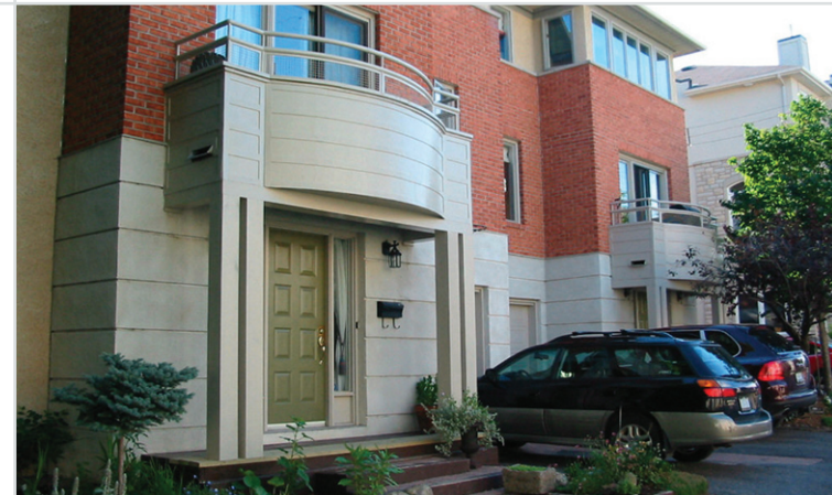
Figure 22: The structural columns and second story balcony articulate the front façade and highlight the entrance to this unit.
