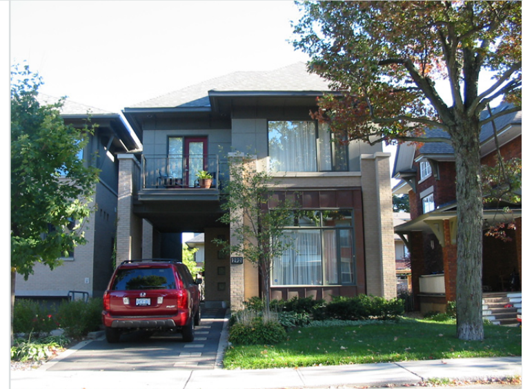
Figure 32: Note the absence of a sloped basement driveway, garage door, and retaining walls to support this infill development; instead here is room for a green front yard and ground-level windows.
