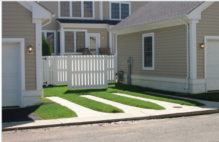
Figure 40: Wheel strips provide a stable base for vehicles; an unpaved driveway allows for increased infiltration.
