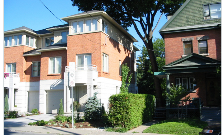
Figure 38: The garage occupies around 50 per cent of the front of these multiple-attached dwellings, and there are no sloped driveways to diminish the streetscape. The infill development also employs successful articulation, visually separating each residential unit from the next.
