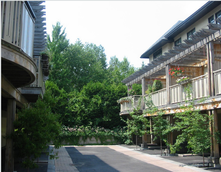
Figure 17: An adequate separation distance between infill blocks (in this example, on a rear private lane) ensures sufficient light, view and privacy for residents. Richly detailed rear balconies and arbours define outdoor amenity areas; complementary screening and planting increase privacy.
