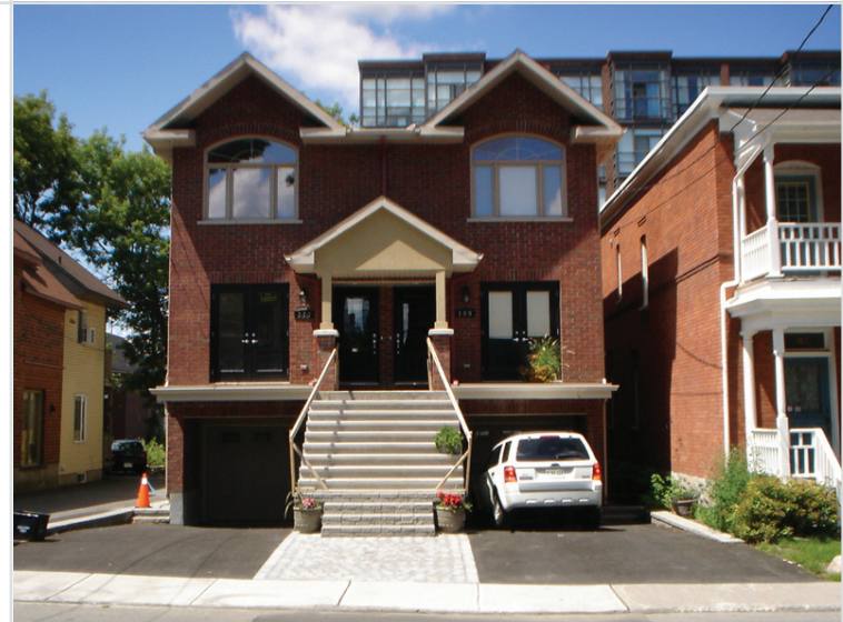
Figure 39: Sloped driveways may be acceptable in cases where the dwelling is emphasized and where the driveway and garage door is de-emphasized. Prominent porches, entry areas, second floor balconies and significant landscaping can help to emphasize the dwelling.
