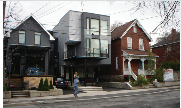
Figure 31: This semi-detached infill unites two different architectural styles. The renovated unit on the left is attached to the contemporary middle unit but reflects the form and character of the existing single-detached red brick home. The contemporary unit adopts the colours of the renovated unit to blend successfully into the streetscape.
