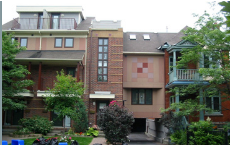
Figure 35: The design of this infill on the left minimizes the impact of car storage by locating shared parking behind the development, internal to the site and accessed through a low entryway.
