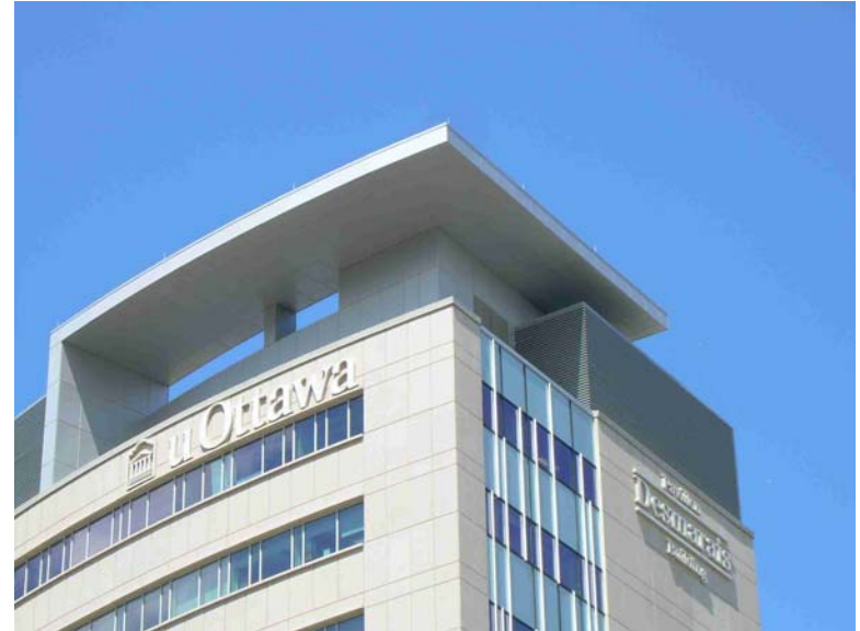
Figure 51: Building utilities are incorporated in the design of the top away from view
