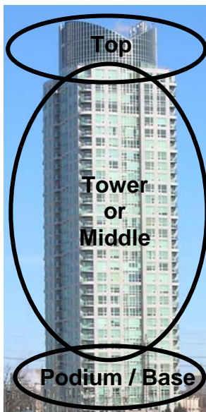
Figure 12: regardless of building style, a high rise has three main components that respond to its function, use and context. Depending on the design style, there may be significant or subtle differentiation in the character or detailing of each of these segments, but they are integrated in the whole of the design.
