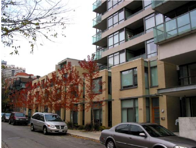
Figure 5: The building base and lower profile buildings create a transition between the high-rise and adjacent development and continuity along the street.
