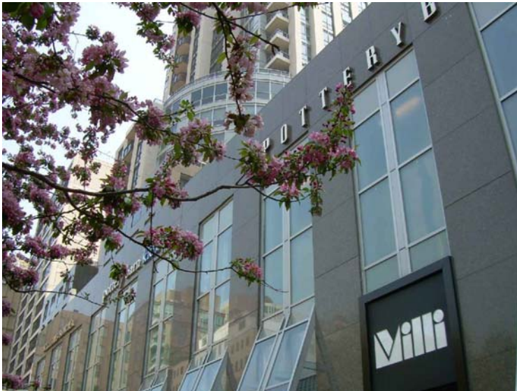
Figure 18: The middle section, stepped back above a podium base, helps minimize the perception of the building's size
