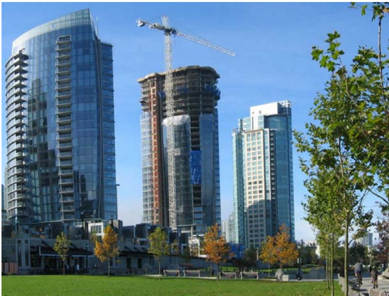
Figure 20: Recent high-rise residential projects in Canada with point tower floor plates of approximately 750 square metres accomplish many of these objectives. Compact commercial footplates are about 1,850 square metres. (Urban Strategies)
