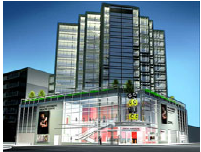
Figure 43: This mixed-use building built on a brownfield site features active solar technology and uses 45% less energy and 45% less water than a conventional building (Windmill Development Group)
