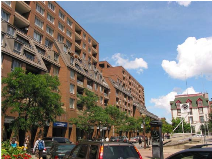
Figure 6: Transitions are created by stepping down using an angled plan defines the building envelope
