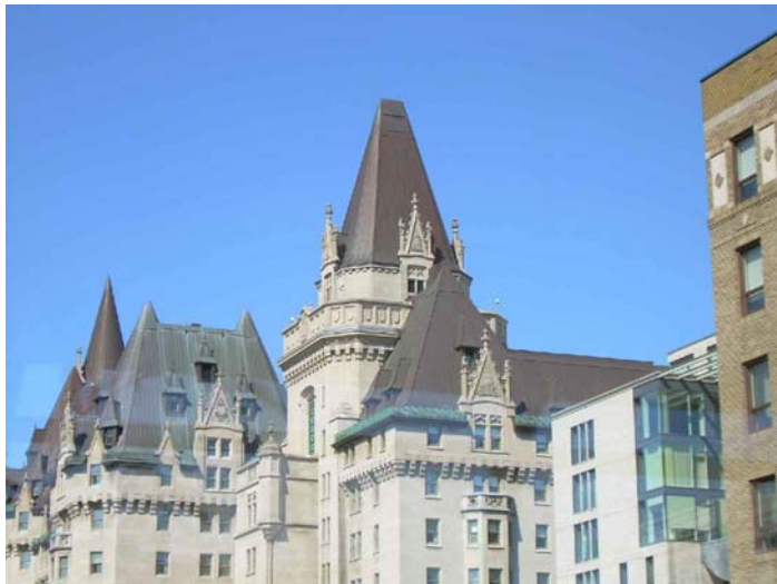
Figure 2: A landmark building demonstrates its place within the community through its design, prominent location or function. It can assist in way-finding or act as a gateway.
