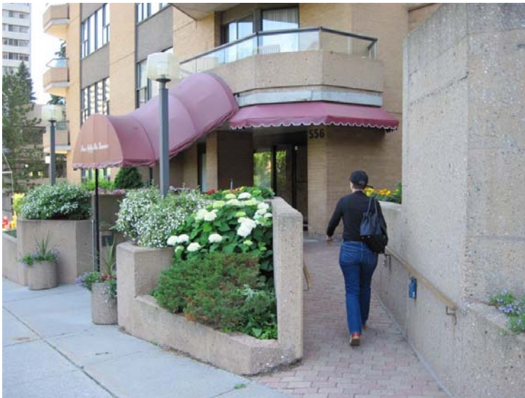
Figure 31: The accessible ramp is well integrated and direct; site furniture and planters are set back and integrated to reduce hazards for those with poor vision.
