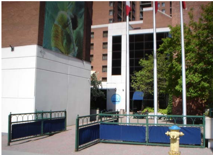
Figure 40: This inner courtyard is open to the public sidewalk
