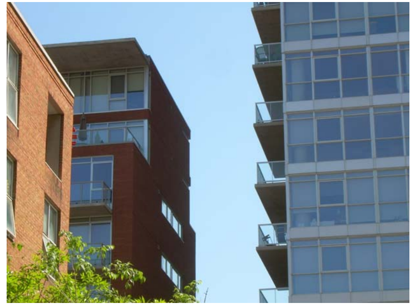
Figure 21: These balconies are oriented to reduce direct views into units of adjacent towers.
