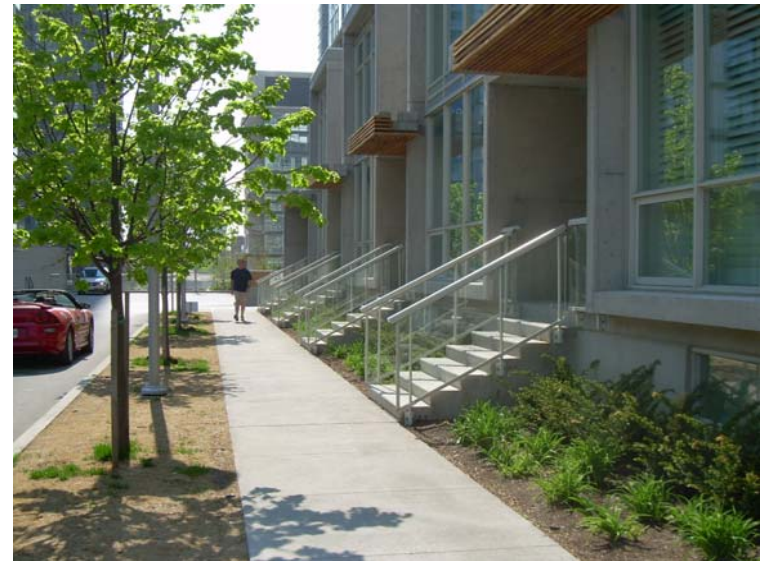
Figure 13: Individual residential units (in the podium base of a high-rise building) are up half a level from the sidewalk and setback with landscaping for privacy. The property line is located where the stairs meet the sidewalk
