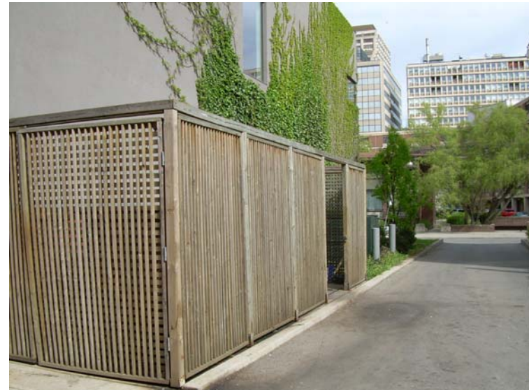
Figure 54: Decorative gates and screens hide utility areas in this service area of the site.
