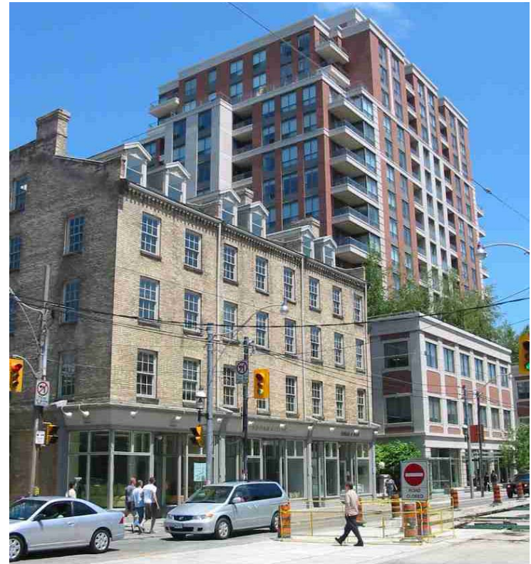
Figure 7: The scale and form of the building podium (with a tower set behind) complements the street scale of the adjacent historic building.
