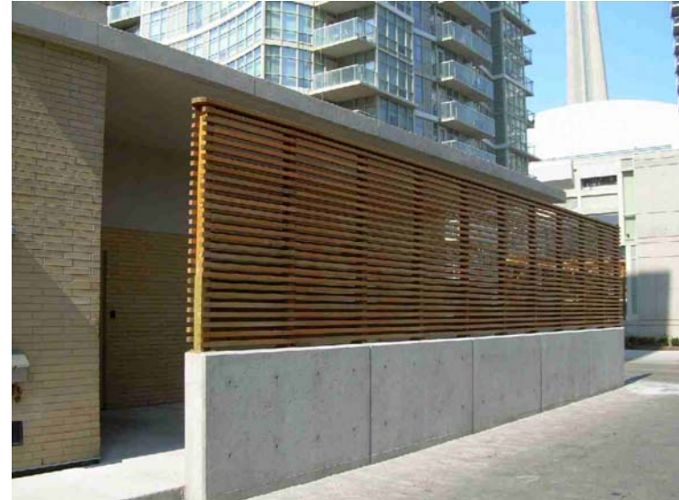
Figure 53: A decorative screen hides the loading area
