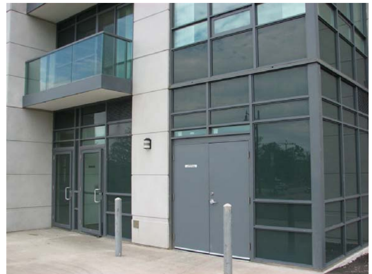
Figure 52: Garbage and recycling is located in a service area behind these doors
