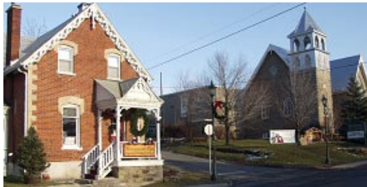
Commercial and institutional buildings along Main Street Photo Courtesy of CSW
