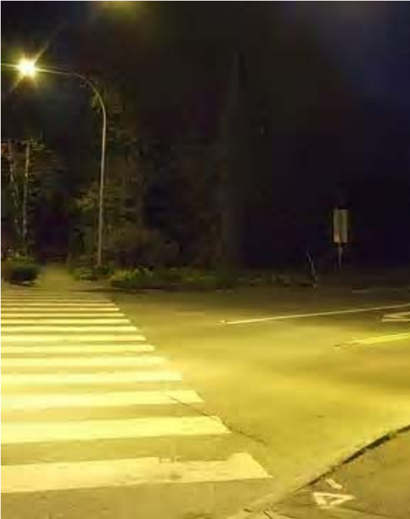
This particular crosswalk has downward lighting from the overhead crosswalk treatment. This helps to highlight the crosswalk location at night but may create “dark” areas at the ends the crosswalk. ( www.flickr.com / photo femme )
