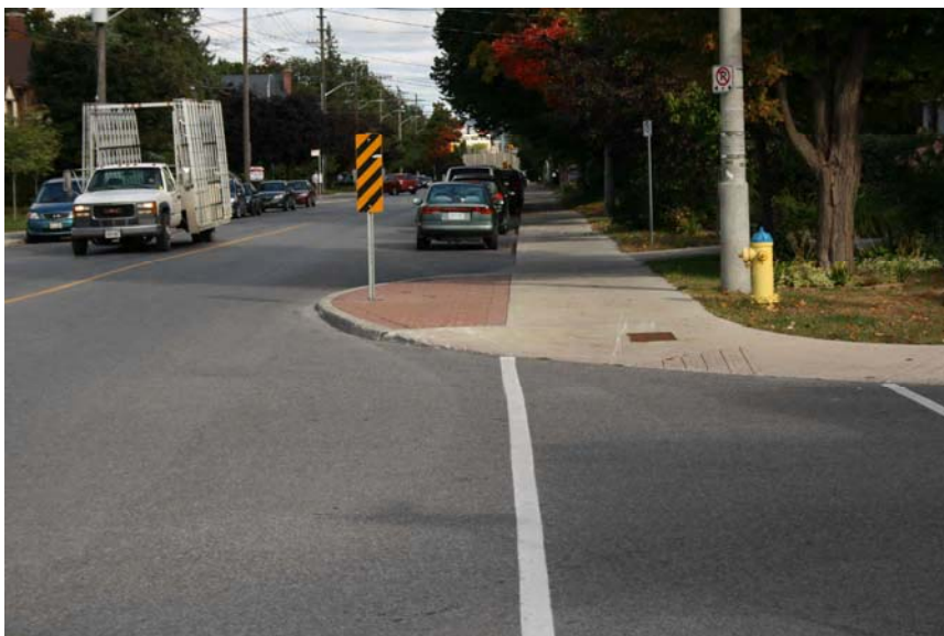
This Holland Avenue curb extension has a curb ramp to transition from the sidewalk to the pavement. Curb ramps must be designed to accommodate wheelchairs, walkers, strollers and so forth. (McCormick Rankin Corporation)
