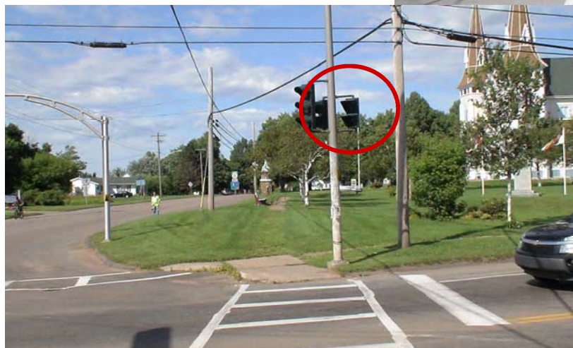
Although not an example in the City of Ottawa, above is a photo of a pedestrian signal head that is not operating. To the left is a photo (at the same intersection) of pedestrian signal heads that are not directed at the pedestrians in the crosswalk and thus are not visible. (McCormick Rankin Corporation)
