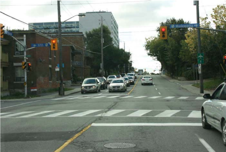
An example of a Bronson Avenue intersection crosswalk with enhanced crosswalk markings. This makes the crosswalk more visible to drivers. (McCormick Rankin Corporation)
