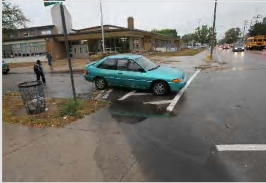
This is an example of a stop-controlled intersection where drivers are required to pull ahead into the crosswalk to see oncoming traffic. Note the standing water that creates a hazard for pedestrians. ( www.pedbikeimages.org / Dan Burden)
