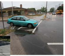
An example of deteriorated pavement and concrete surfaces is shown at left. The result of poor maintenance is shown above where standing water is located in the crosswalk. These types of conditions can be a hazard to pedestrians and increases agency liability. (www.pedbikeimages.org / Dan Burden / McCormick Rankin Corporation)
