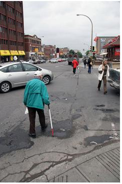
In the above photo, the deteriorated pavement markings make it difficult for drivers to detect its presence. (www.pedbikeimages.org / Dan Burden)
