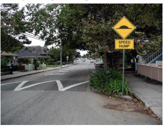
Speed humps and tables are often used to help reduce vehicle speeds in advance of pedestrian crossing areas. (Dan Burden / McCormick Rankin)
