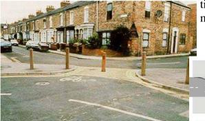
The above photo illustrates a diagonal diverter with removable bollards for emergency access. To the right are examples of the four basic types of traffic diverters. (FHWA University Course on Bicycle and Pedestrian Transportation)
