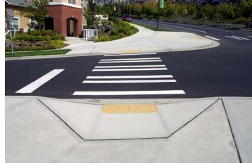
An example of a curb ramp to provide an adequate transition between the sidewalk and roadway. This particular installation has a texturized and coloured pad at the bottom of the ramp to assist special needs pedestrians but its use is not standard practice in Ottawa. (www.pedbikeimages.org / Dan Burden)
