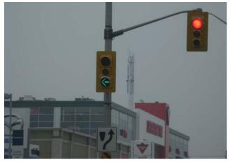
An advance left turn phase for vehicles allows the majority of turning vehicles to clear the intersection before pedestrians enter the crosswalk, limiting the potential for conflict. (City of Ottawa)
