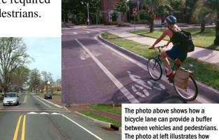
The photo above shows how a bicycle lane can provide a buffer between vehicles and pedestrians. The photo at left illustrates how bicycle lanes help narrow the travel lanes and may help to reduce vehicle speeds. (www.pedbikeimages.org / Dan Burden)
