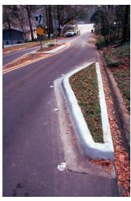
Chicanes are much like midblock chokers, however they are offset to force drivers to shift their driving path. The result is a narrow roadway and slower vehicle speeds. Careful design is required when considering chicanes. If they do not extend out from the curb far enough or have a large space between installations they can be ineffective. Conversely, they should be designed to preserve enough lateral space to permit shared lanes to accommodate cyclists.
