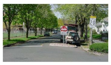
This is an example of a partial intersection closure that prevents vehicles from entering the street. As a note, the signage illustrated here is not consistent with the practices of the City of Ottawa for this type of treatment. (www.pedbikeimages.org / Dan Burden).
