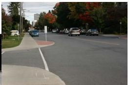
The Figure above shows a curb extension on Holland Avenue in an area of on-street parking. (McCormick Rankin Corporation). The Figure at left is an example of how a curb extension helps to make a pedestrian more visible by locating the refuge area closer to the travel lane. (www.pedbikeimages.org / Dan Burden)
