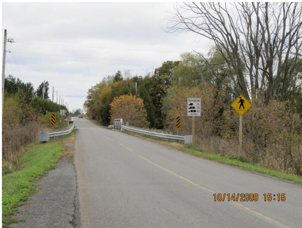
Looking west at bridge
