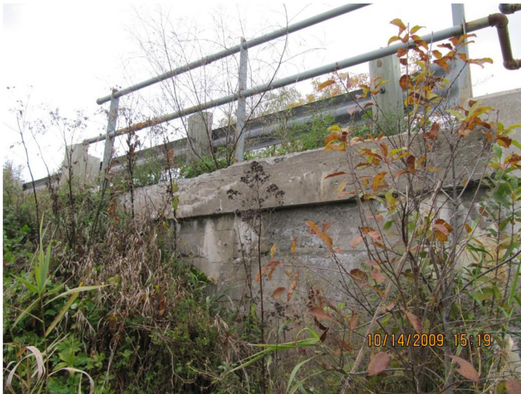
South west wingwall
