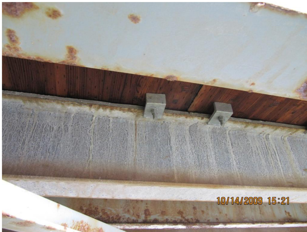
Detail of steel stringer and deck clip
