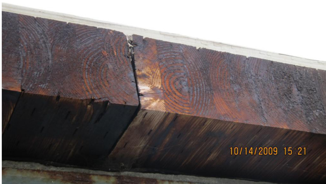
End view of timber deck (south side)
