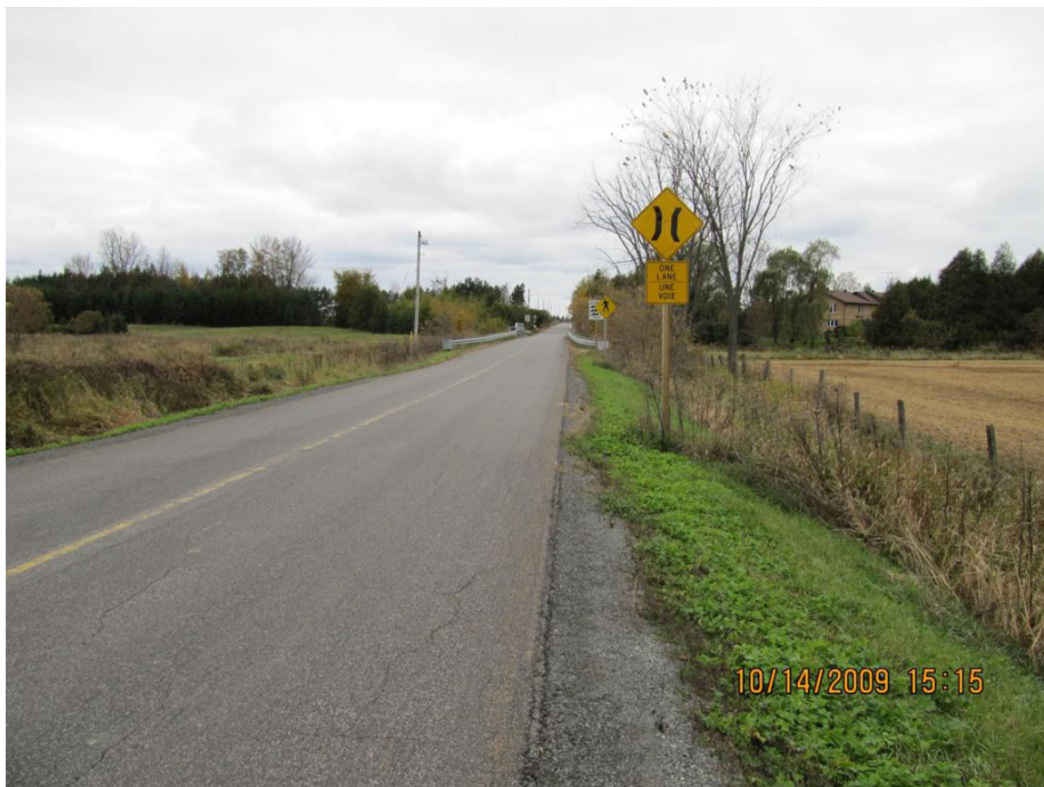
Looking west from east approach
