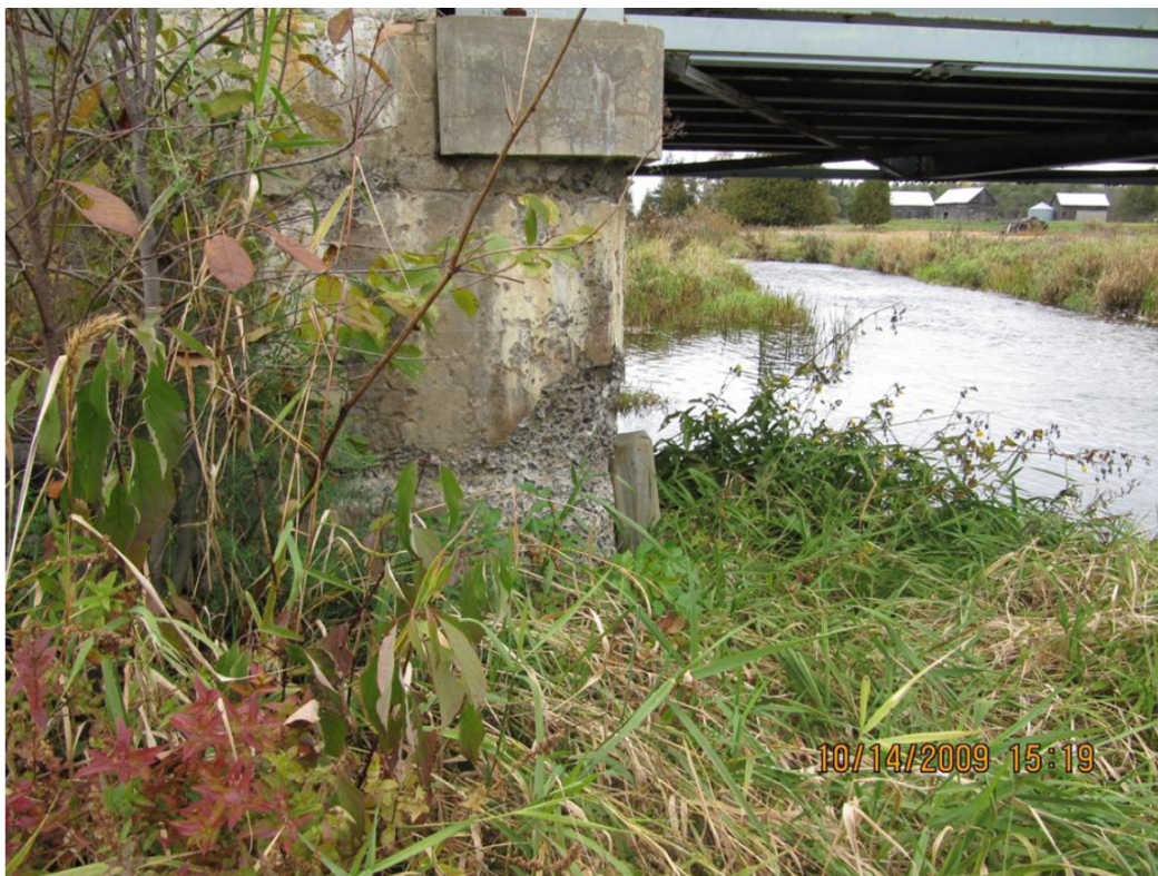
South end of west abutment
