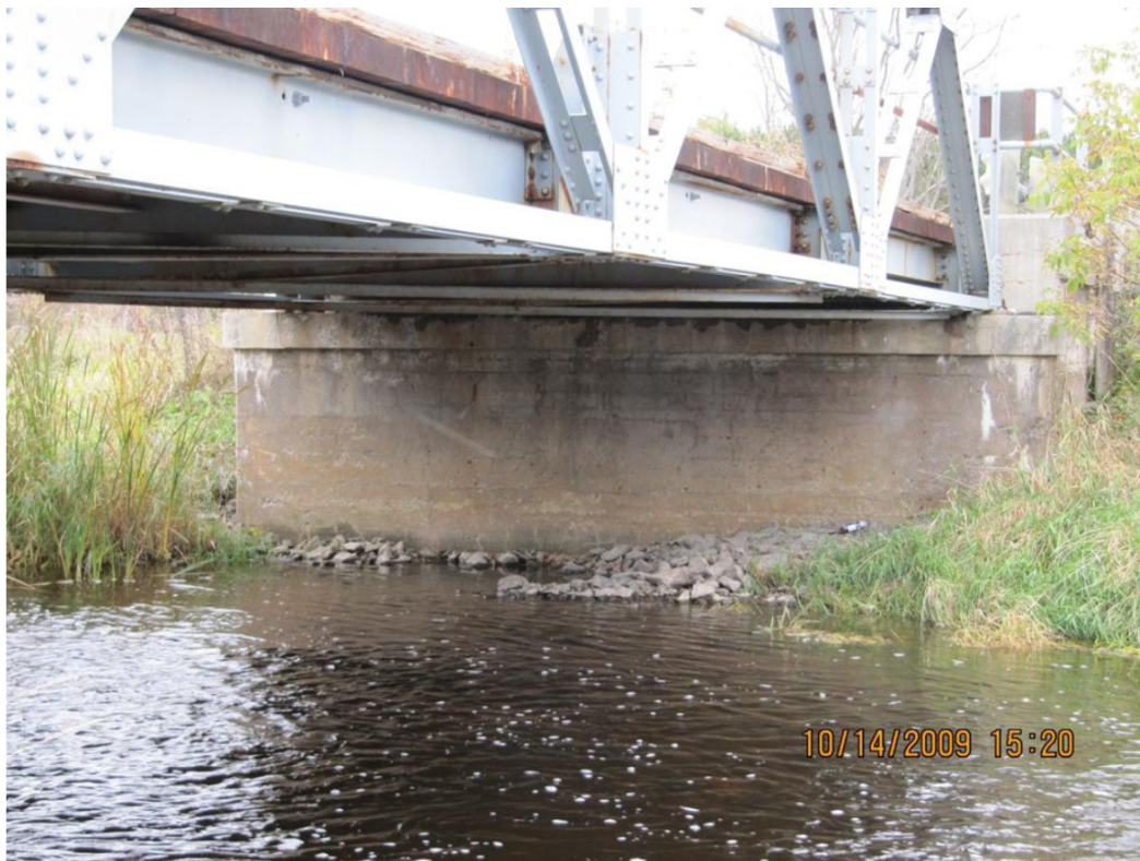
View of east abutment
