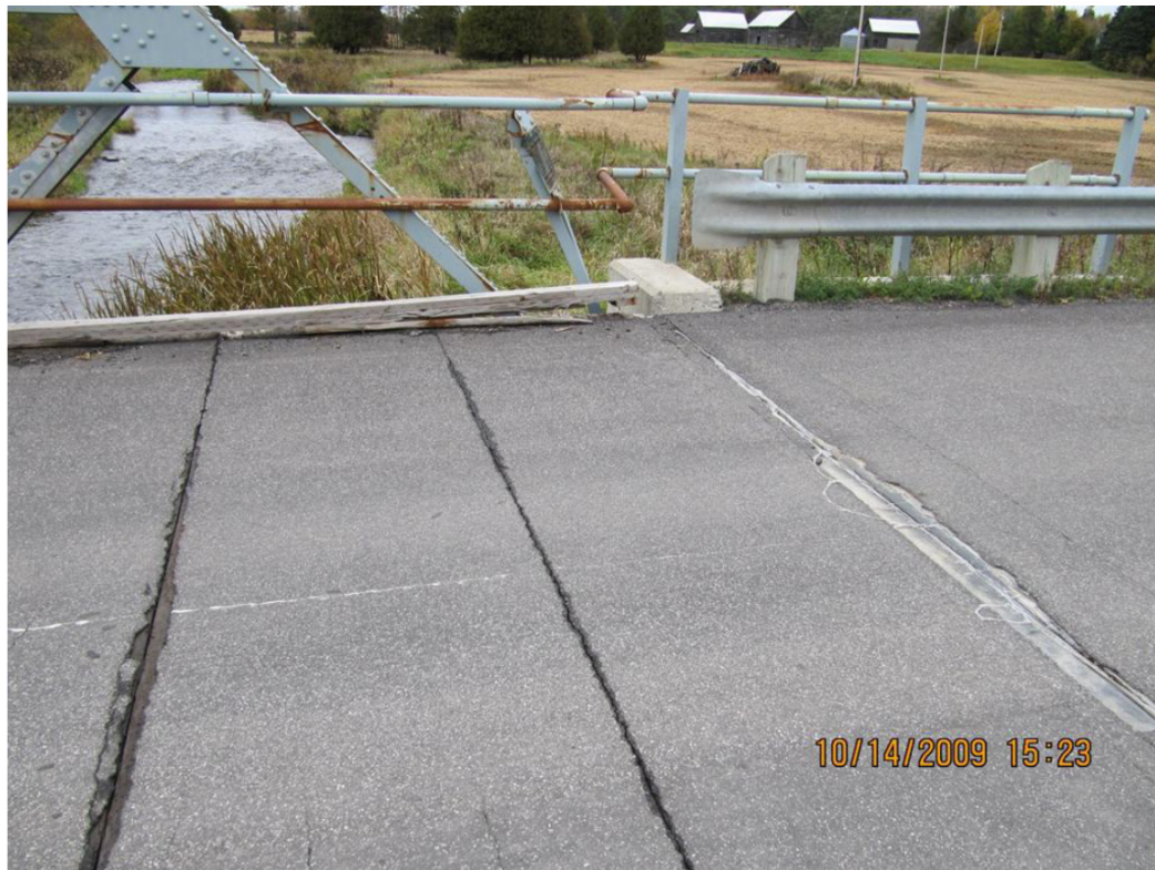
View of deck, north curb and barrier, east expansion joint
