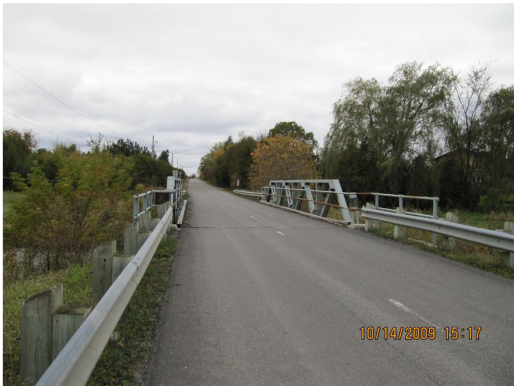
Looking west at bridge
