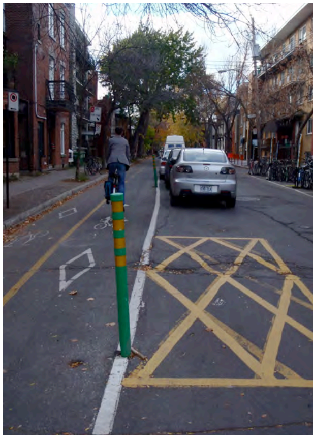
Figure 8. Painted line and posts as separators
