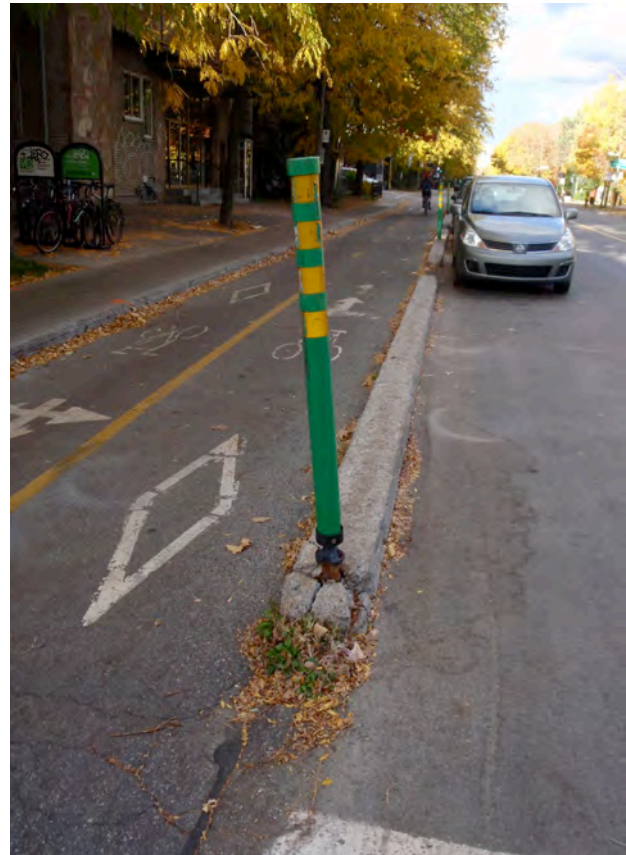
Figure 9. Permanent concrete divider as a separator
