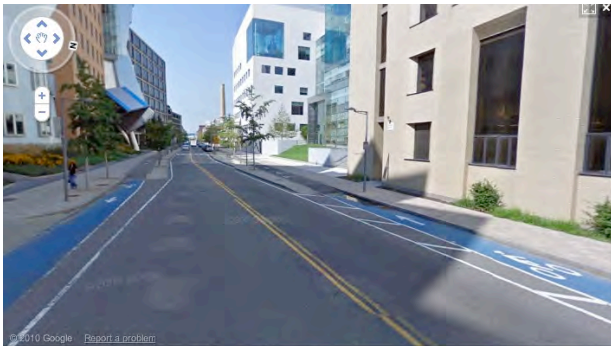
Figure 5. Transition from segregated to conventional bicycle lane, Vassar Street, Cambridge, MA
