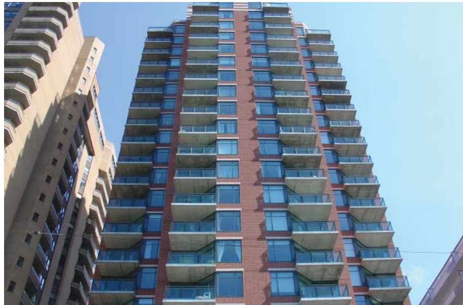
The "Laurier" residential tower
