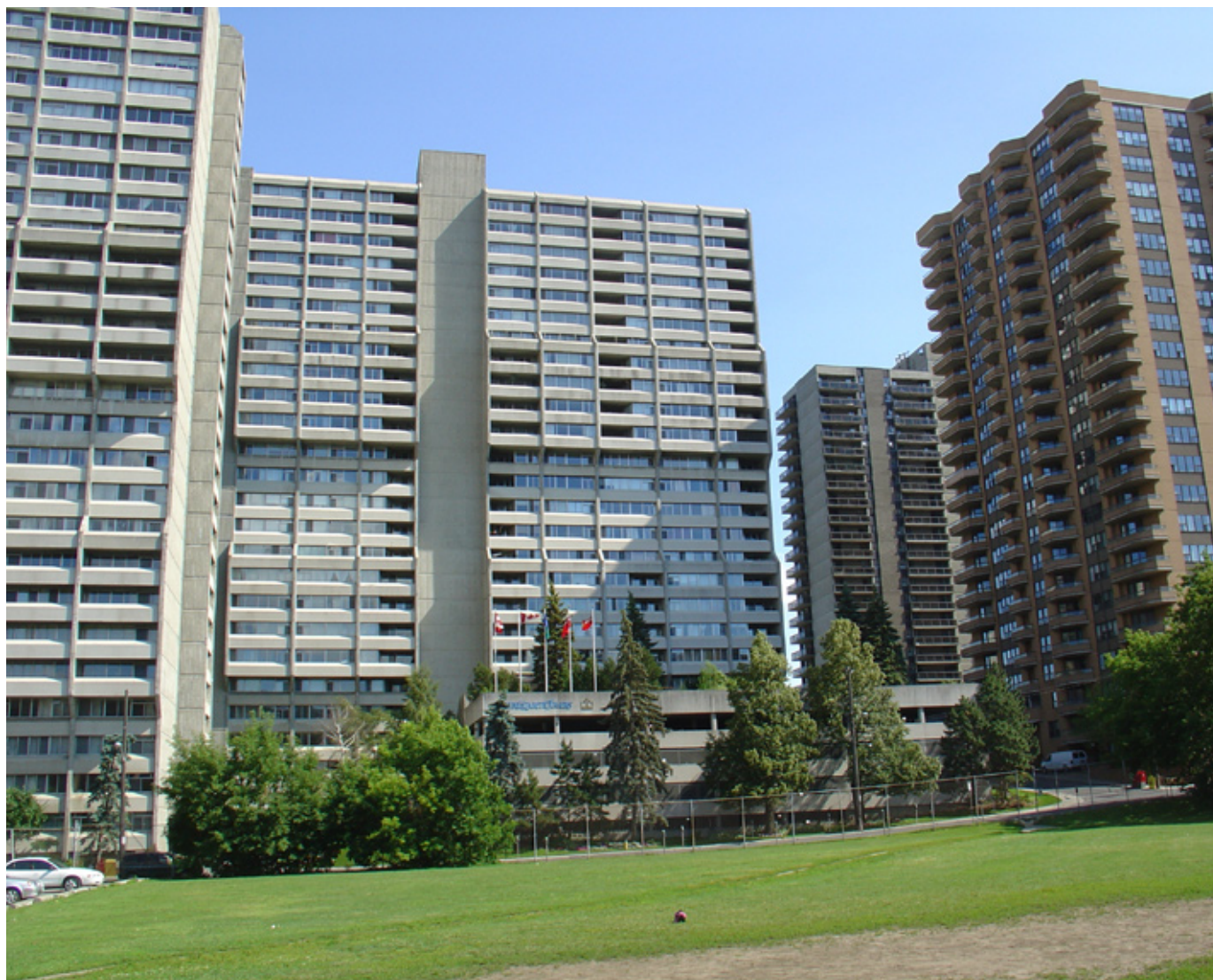
Changing past practices: large building floorplates with little space in between. Escarpment District, Ottawa.
