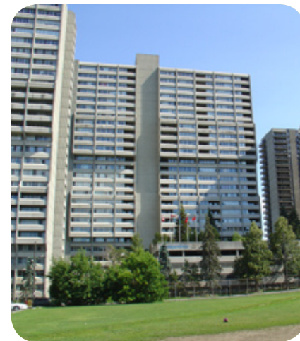
Queen Elizabeth Residential Towers
