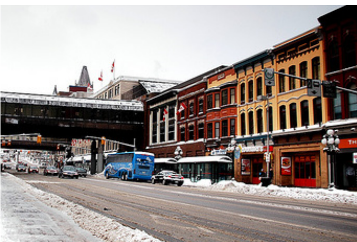
Existing bus shelters along Rideau Street.
