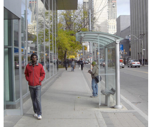
Narrow Transit Shelter -Toronto, Canada
